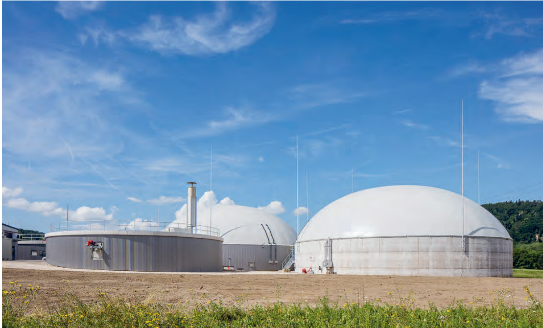
The biogas plant in Henniez, built and run by Groupe E Greenwatt, is the largest of its kind in Switzerland.
