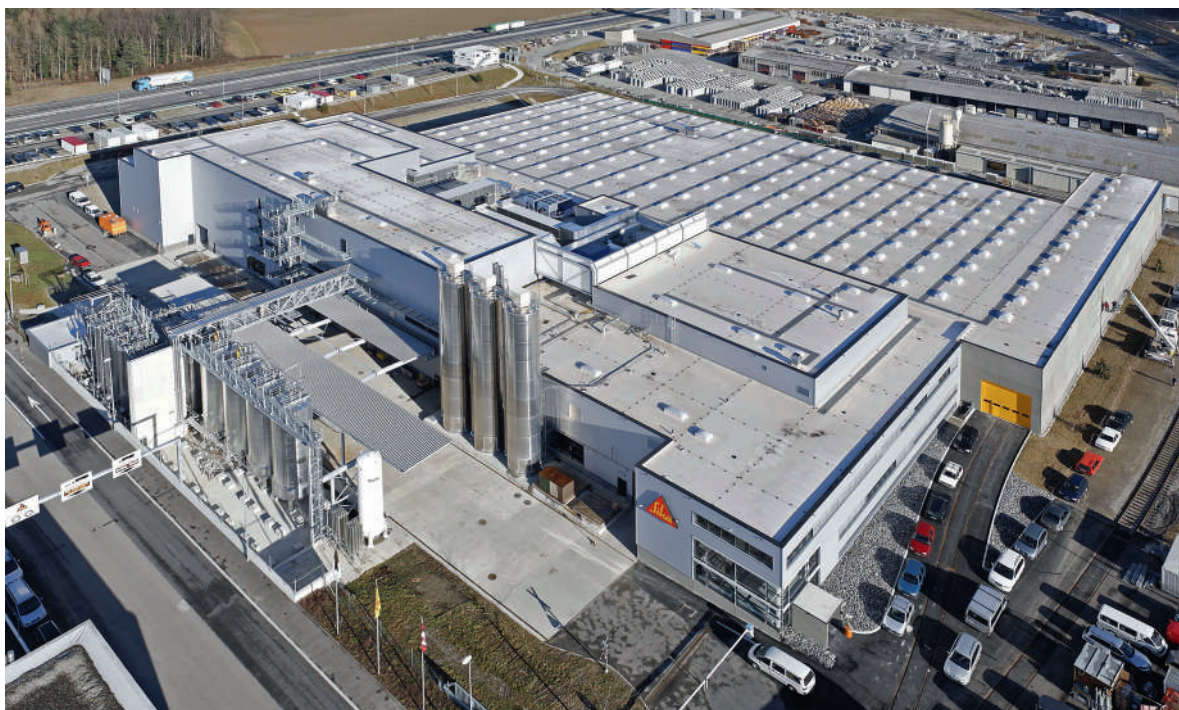
When it comes to efficiency, Sika's production plant in the canton of Fribourg is a role model for many of the group's 90 subsidiaries around the globe.
